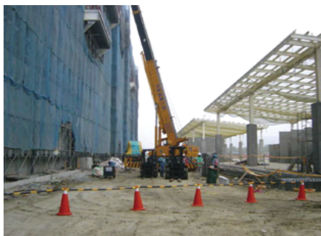
● 吊裝區防護警戒 Work area security
